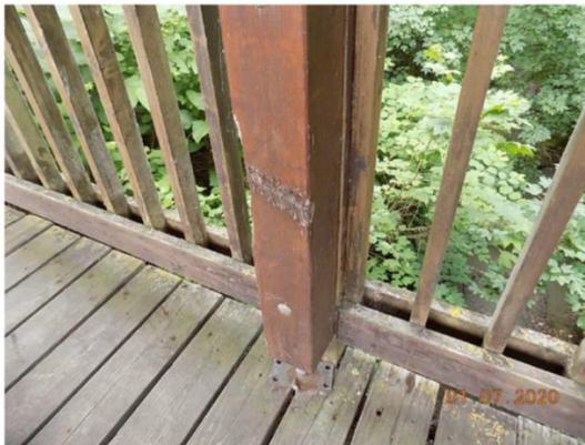
2020\_H\_STÜTZE DES DACHES\_ANPRALLSCHADEN
